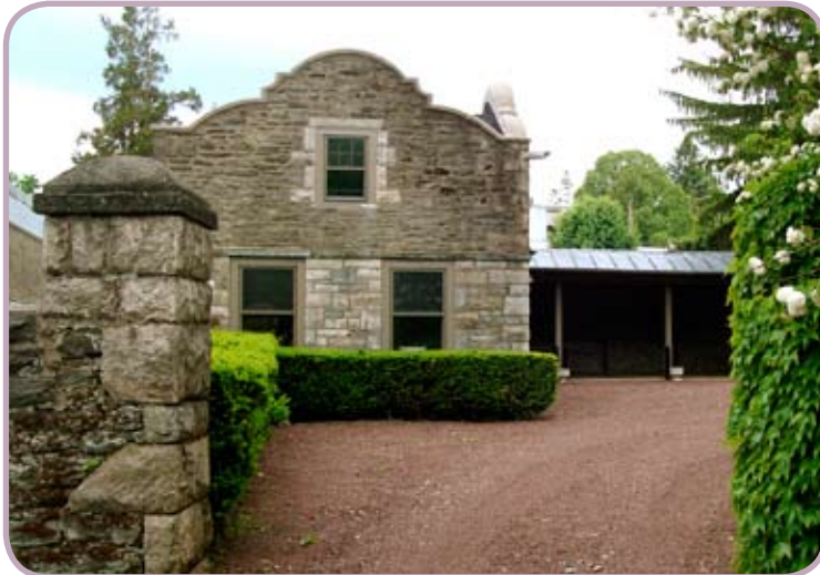
T4 - Crushed Stone Parking - Chestnut Hill, PA
