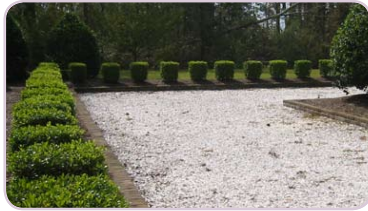
T3 - Crushed Shell - Edenton, NC
